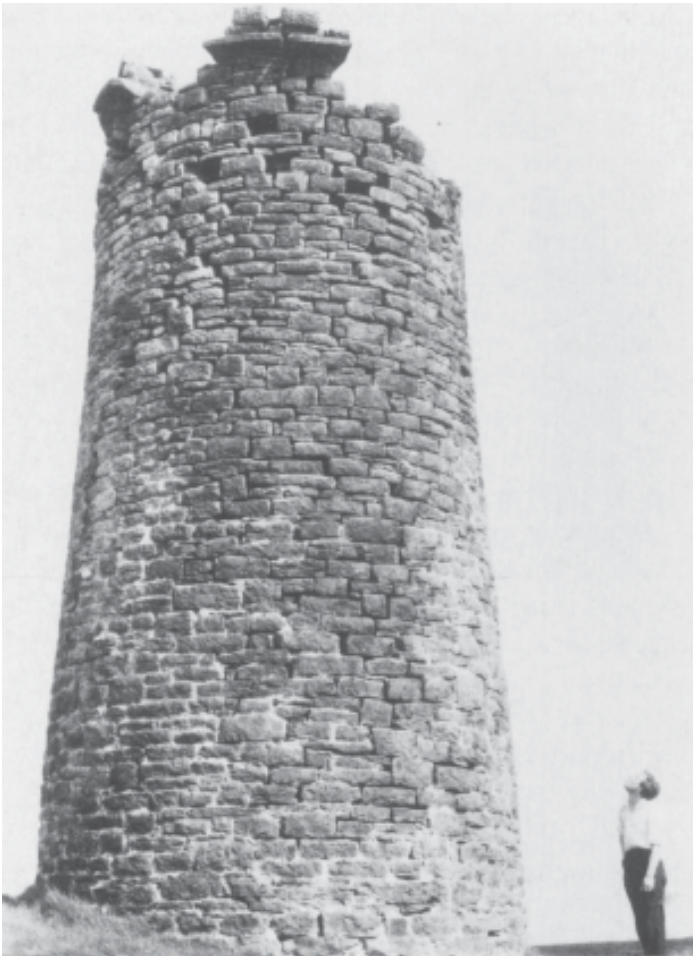
PLATE III. The smelt mill chimney.
