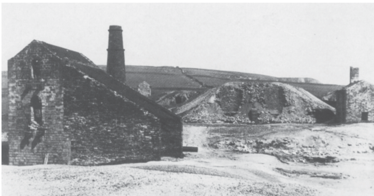
PLATE I. Cononley engine house and shaft, c1905.
