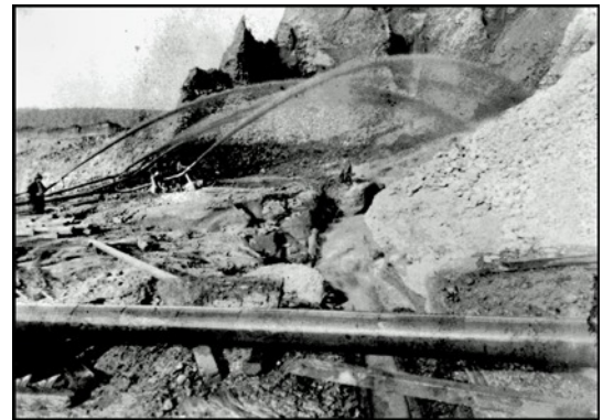
Fig 06 A photograph taken at the height of the gold rush on the Yuba River, showing prospectors firing powerful streams of water at the gold-bearing hillside. Note the metal pipe in the foreground, which brought water many miles across country to meet the huge demands for water.
