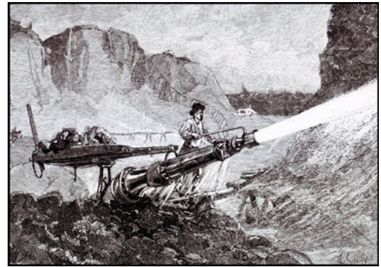
Fig 05 A sketch shows the important details of a ‘monitor’; that is, the counterweight, the powerful stream of water and the handle for aiming while loosening auriferous gravel.
