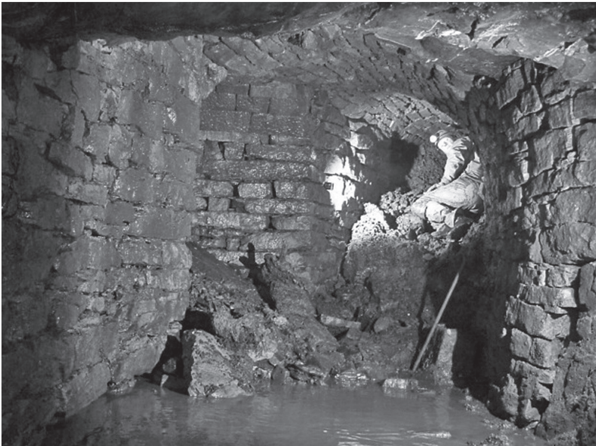
Figure 8. The fall in the horse level which prevents access to the sump top. The tailrace, taking water from the wheelcase, is on the left. [D. Carlisle, 2008].
