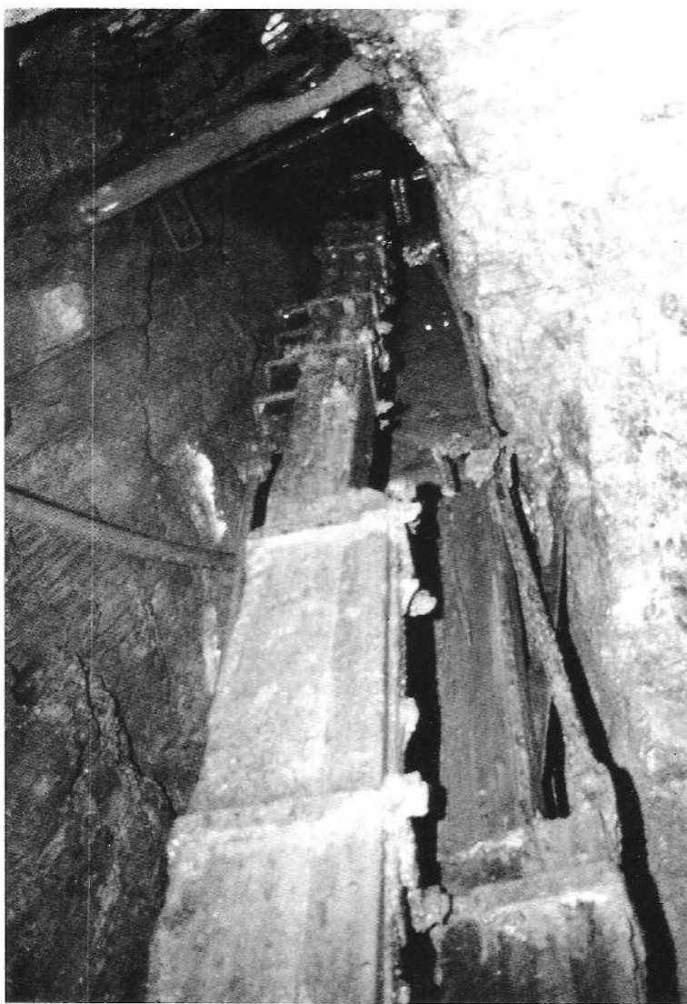
PLATE XVIII. A view up Engine Shaft from adit level, showing two massive timber pump-rods and a collapsed iron rod on the left. A fourth rod, also timber, is obscured. (R.A. Southwick).
