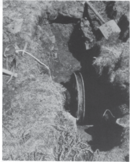
Return wheel in working position
