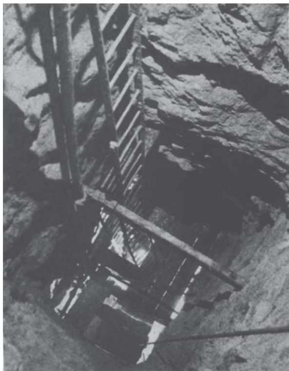
PLATE V. LADDER ROAD IN THE HAULAGE-WAY NEAR ADIT LEVEL. (PHOTO: R.H.B.)
