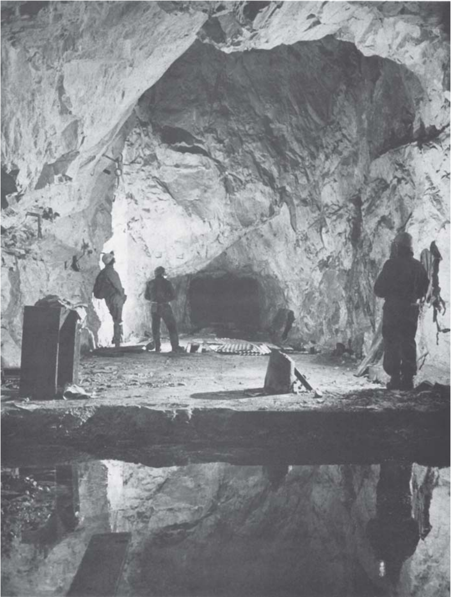
PLATE I. GREENSIDE MINE. ENGINE ROOM AT COLLAR OF SMITH'S SHAFT, LUCY TONGUE LEVEL. THE SHAFT IS BENEATH THE CORRUGATED SHEETS (CENTRE) AND IN THE FOREGROUND IS THE FLOODED WINDING ENGINE EMPLACEMENT. (PHOTO: R.H.B.)
