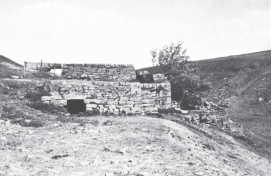
Plate 1. Shaft Top View looking north May 1980
