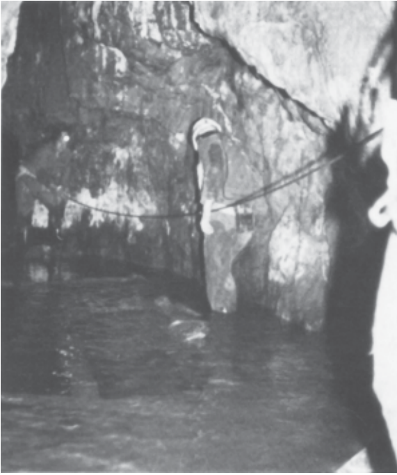
Flooded stope and timbers. Candle soot marks may be seen on the wall above the centre person.
