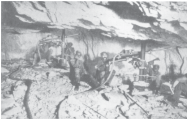
Fig. 13. "Dry" compressed air drills being used in a South African gold mine (c.1905). Experience with such drilling equipment led to the realisation that dust was the cause of the high mortality from miners' disease on the Rand and elsewhere.
