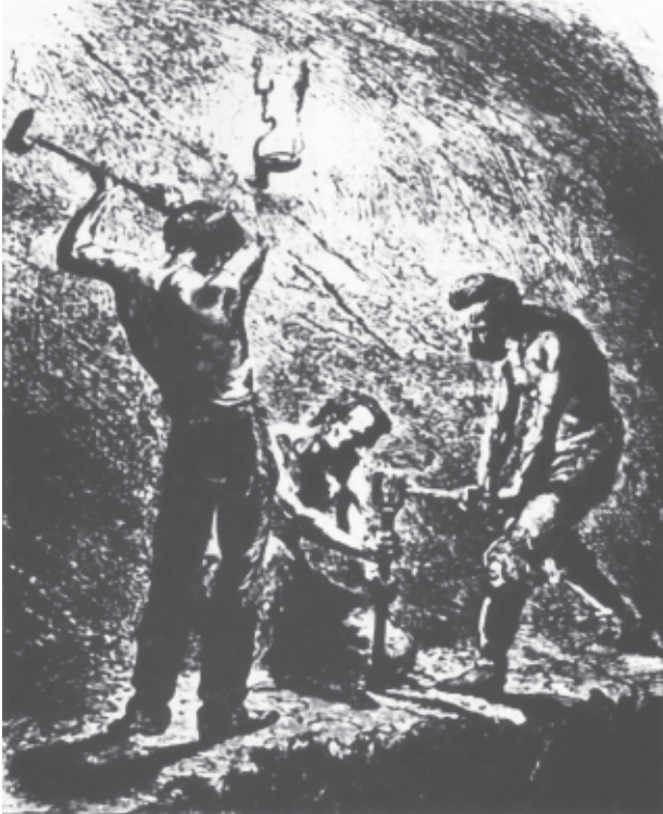
Miners boring a hole downwards by hand. Dust was produced by many underground activities, especially boring holes. Hand boring was done by one, two or three miners, horizontally as well as upwards and downwards. (From Simonin: Underground Life. 1869)
