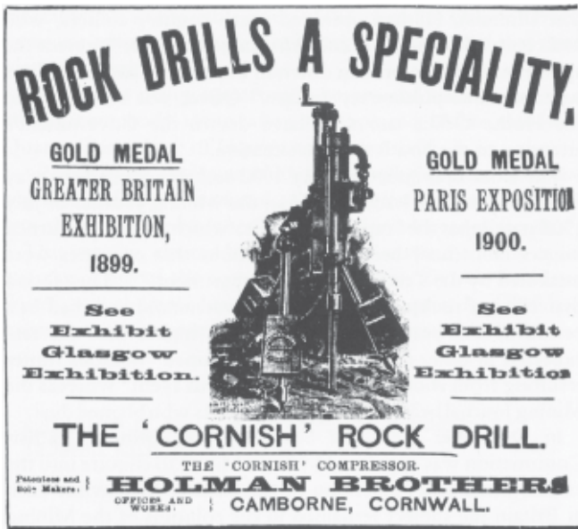
Fig. 14. Advertisement in the 1903 Mining Journal for one of the “dry” compressed air drills which increased dust levels so much that a major increase in the death rate from lung diseases took place.
