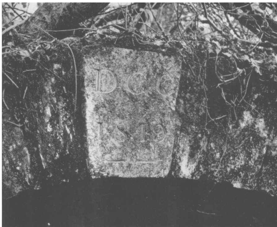
Plate III. The inscription “D.G. C. 1819” on the keystone of an arch which straddles the Devon Great Consols leat, near to the site of one of the huge pumping wheels. As far as is known, this remains the only extant field reference to this huge Victorian enterprise. (SX 427725).
