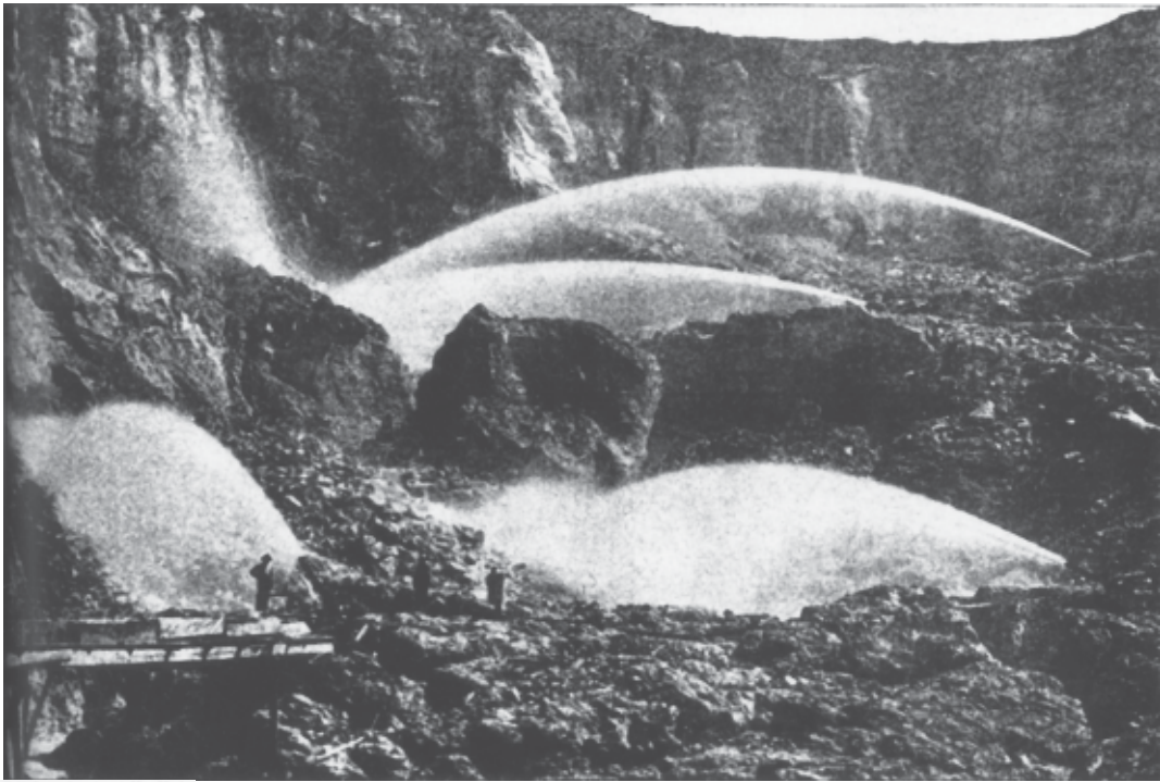
Fig. 5. The colossal thirst for water, occasioned by 'hydraulic'ing', required leats of large capacity, never equalled in Britain. Some idea of water consumption can be gained from this illustration of a section of North Bloomfield mine, Nevada. (after Lock).
