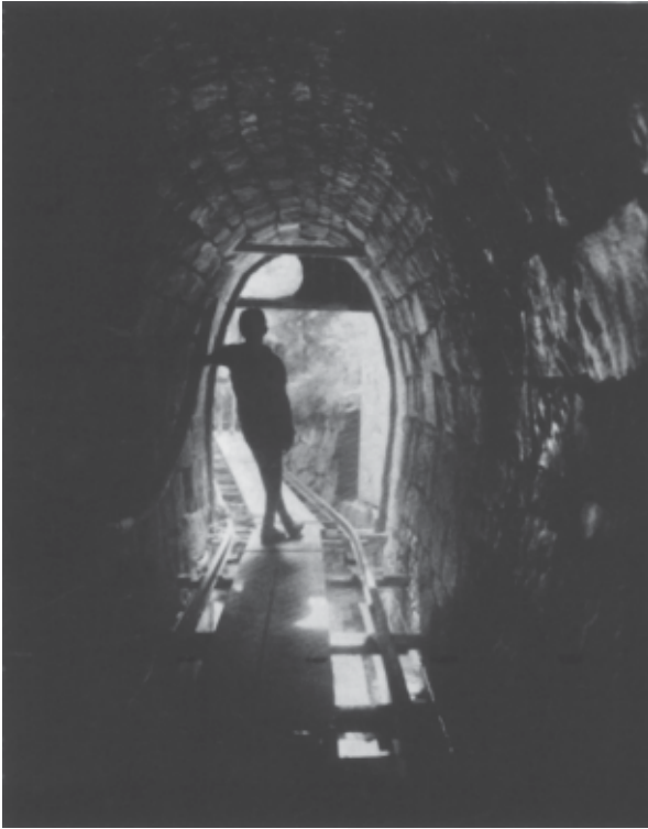
(left) Plate IX. Complete with rails supported above water, the Schulte Wasserlauf conveys a rapid stream through a hillside to modern turbines near Bad Grund, Harz.
