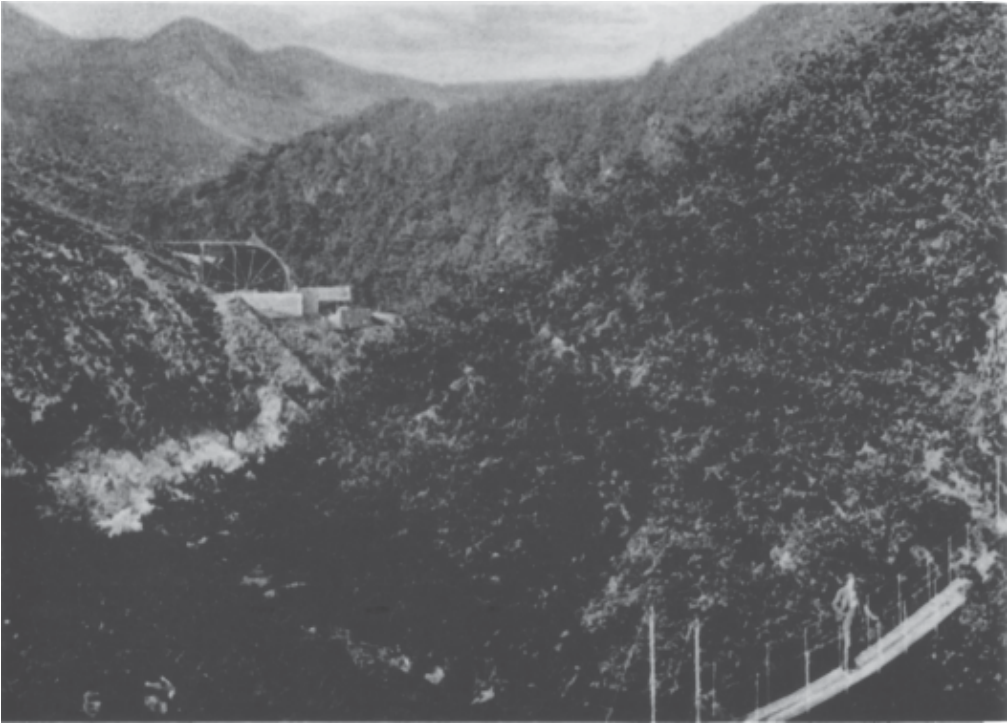
Plate IV. Tucked away in a rocky gorge, Temple Mine, mid Wales, required a considerable 'head' of water for its crusher wheel (and pumping wheel, out of sight beyond), so a leat tapped the river some considerable distance upstream. Long stretches of launder carried the channel parallel to the gorge and down to the mine. Parson's Bridge in the foreground.
