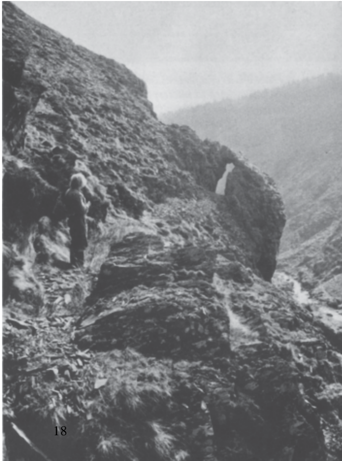
Plate V. Opposite Castle Rock, the Dyfngwm leat, mid Wales, contours the steep hillside, through an arch of rock. Just beyond, the channel was possibly laundered over the outcrop of the lode.
