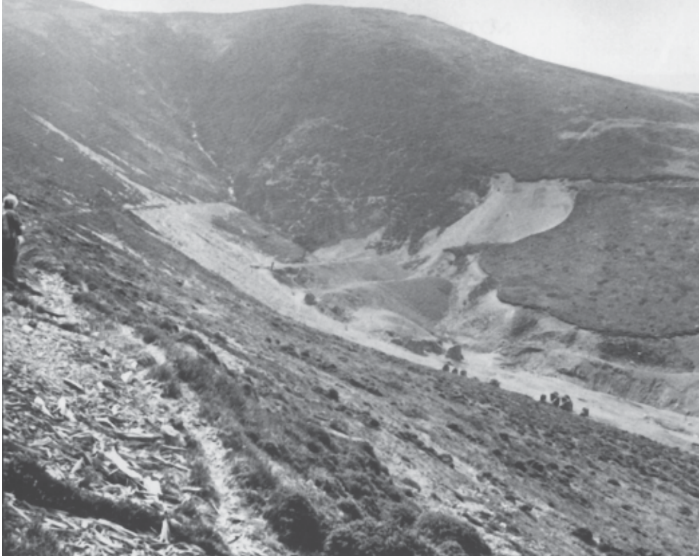
Plate VI. Water for the Cwmbyr Mine, mid Wales, was obtained from two impressive leats. Designed to intercept many of the small streams and running below steep crags, their dried up beds provide a splendid approach to this remote working. (SN 786946).
