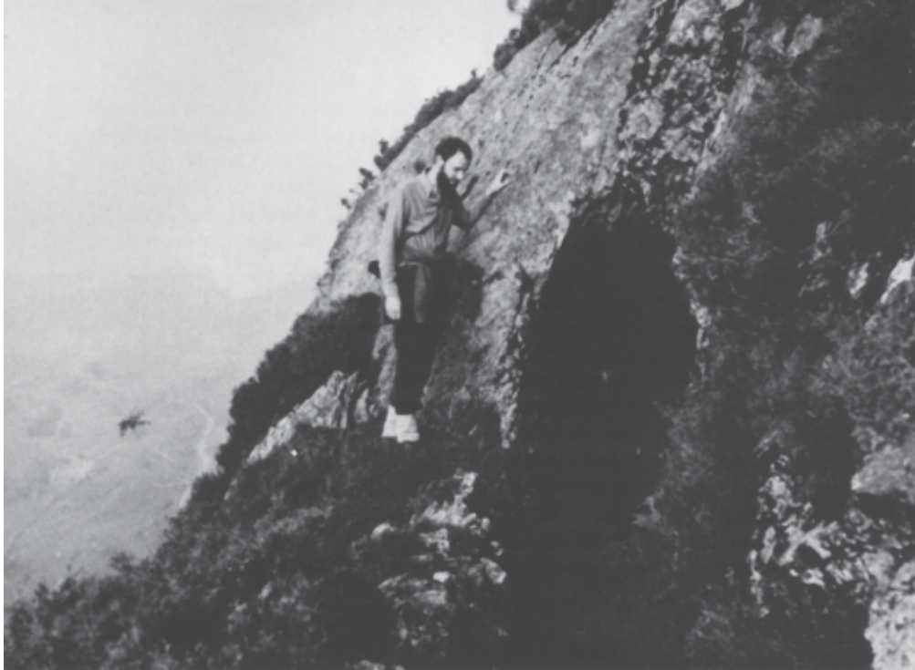
Plate VII. One of the tunnels on the leat high above the workings of Drwsycoed copper mine, North Wales. There is almost a sheer drop on the left into the valley below. (SH 543533).
