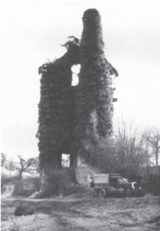
Plate III. Clay's enginehouse, Vale of Towy Mine, near Carmarthen 1957. This fine building housed a 50 inch Cornish engine, set to work in 1852. It was sadly demolished recently, it is said, when the owner was refused planning permission to turn it into a house.
