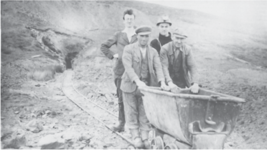
Plate II. Clearing the adit at Esgairmwyn, 1949. An attempt by George Hall (wearing helmet) to gain access to a blende lode shown on old plans. Bad ground brought the venture to a stop. The level is now quite run in.
