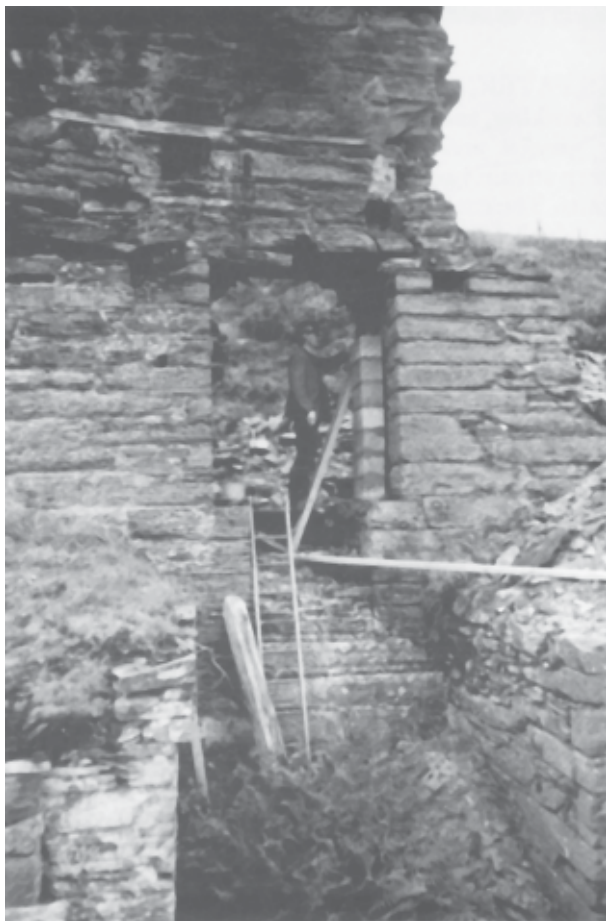
Plate V. Frongoch Mine, near Devil's Bridge, 1982. Emergency measures were taken to prevent imminent collapse of the bob wall, which is still standing. The site has since been scheduled, but paradoxically this would no doubt have prevented such treatment being carried out.
