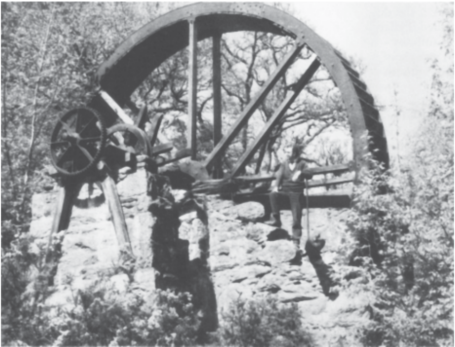
Plate IV. Trecastle Mine, near Conway, 1970. A splendid example of a waterwheel for pumping and winding. The purpose of the spur gear is not certain. The wheel was taken down some years ago and its fate is obscure.
