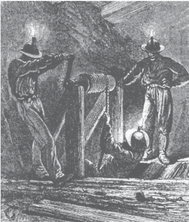
Figure 2. Winze shaft in an old Cornish Mine.
