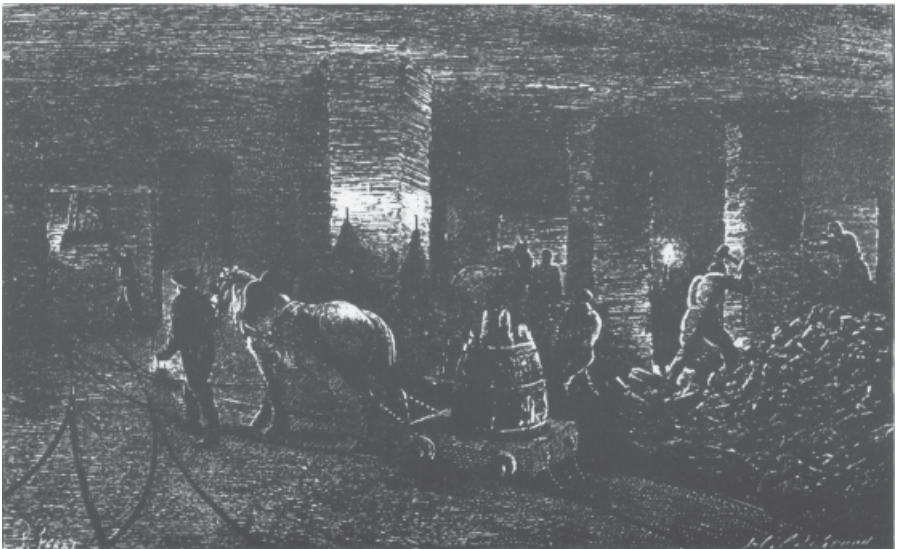
Working coal in the thick coal seams of South Staffordshire.
