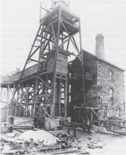
Robinson's Shaft showing 80 inch pumping engine house.
