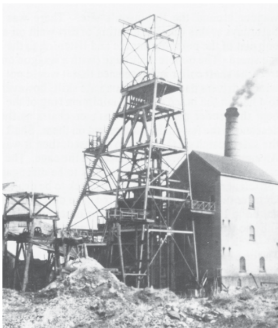
New Cookskitchen Shaft showing 90 inch pumping engine house.
