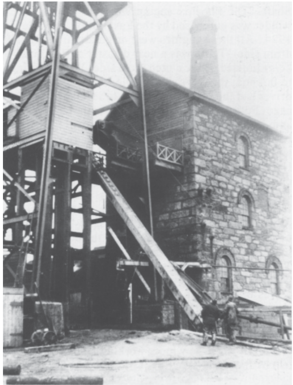
A new top main rod being hauled into place by the capstan engine at Robinson's Shaft.
