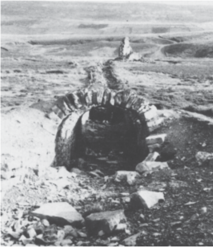
Plate II. Upper section of Surrender flue and old chimney (from above) (S. Bassham, 1992).
