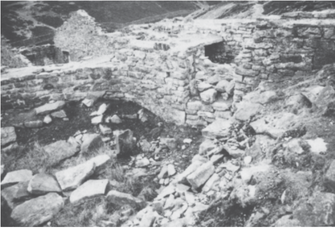
Plate V Cleaning door in Surrender flue and settling area (S. Bassham, 1992).
