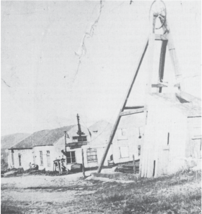
The Wilson Mine in the 1920s. The winder was electric powered, but the original plant had a 30 HP Fowler steam winder. The air compressor installed in 1909, was at the back of the windowless building on the right.
