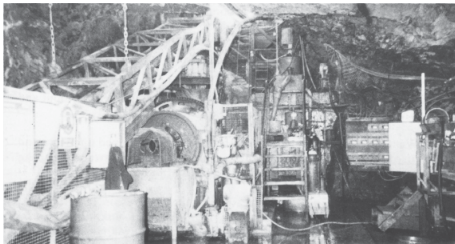
PLATE 4. View of the underground mill. The principal features are (1) conveyor from jaw crusher, (2) gyratory crusher, (3) rod mill, (4) screen, (5) 12" Knelson concentrator, (6) 7.5" Knelson concentrator and (6) Wilfley table. (S.C. Dominy, May 1996).
