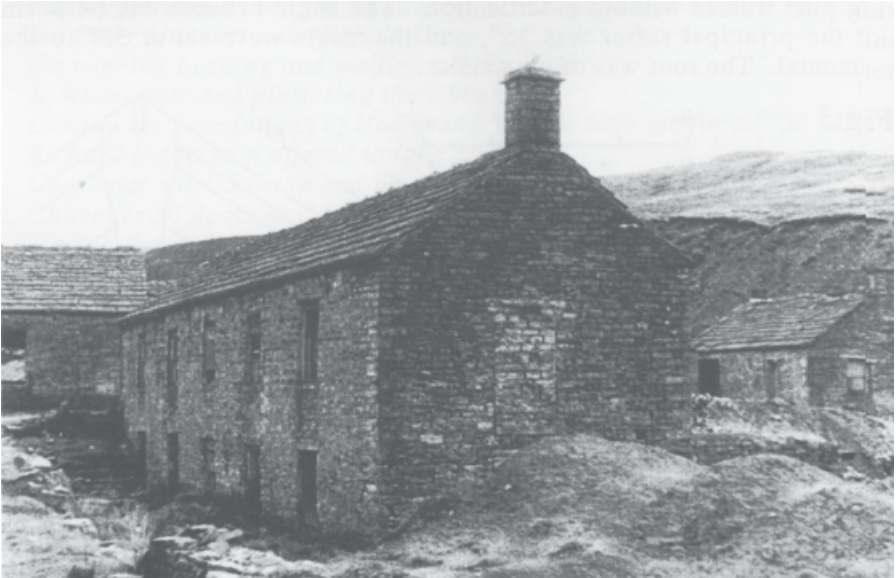
PLATE I Building No.4 (buildings No.2 to the left and No.3 to the right).
