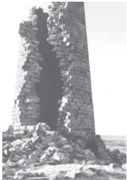
Plates II & III The small chimney after the collapse (Fairbairn, 1994).
