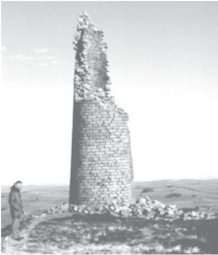
Plates II & III The small chimney after the collapse (Fairbairn, 1994).
