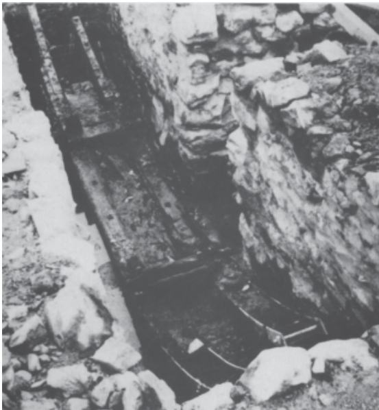
Plate 2. A fragment of the water-wheel partially exposed in a repaired wheel-pit. Tailrace midway on the right.
