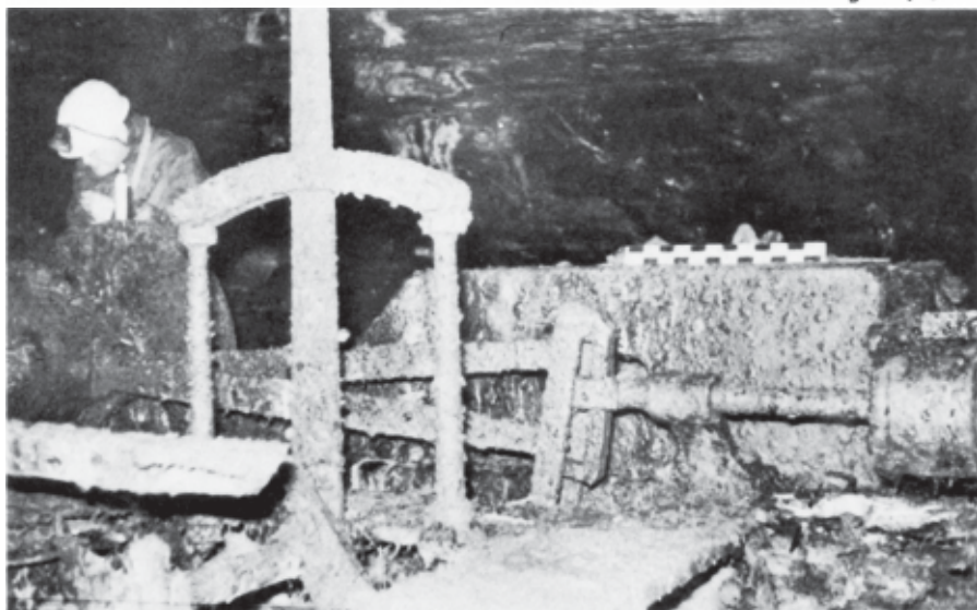
Fig.2. ECCENTRIC VALVE GEAR WITH CHANGE LEVER AND FOOTBRAKE IN IMMEDIATE FOREGROUND
