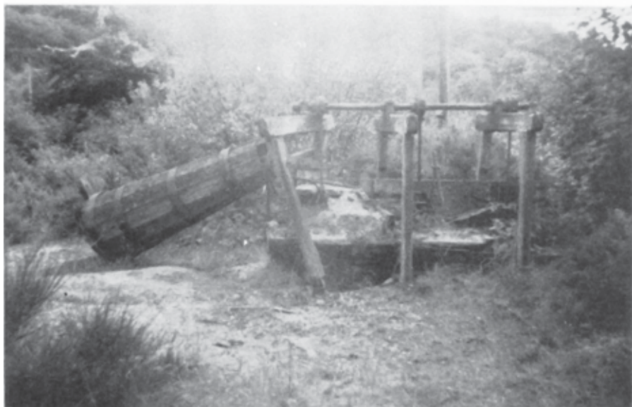
Fig. 2. TROMMEL, BLACK TOM SHAFT. AUG. 1967 PLATE. 11. Photos. R. V. Davis.
