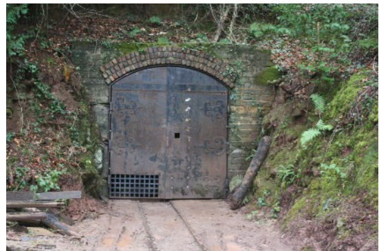
Photo:- Mine door with grill to allow excess water to escape
