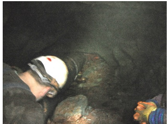
Photo:- installing pipe at furthest zone of weak rock
