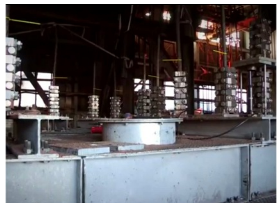
Photo :- Shaft cover structural box with I beams mounted on top and rope clamps in position.
