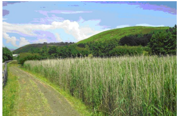
One of the 16 reed beds at Taff Merthyr passive mine water treatment scheme
