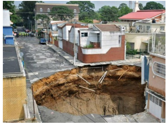
A sinkhole in the North East of England which appeared over night.
