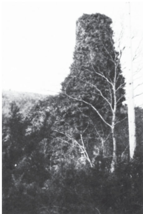
Plate V. Frank Mills. The ivy-encrusted chimney and engine house which stood at the collar of the main shaft and which contained the 60" engine erected in January 1855, sold for scrap in 1880. Like the engine house at Wheal Exmouth, on porter's shaft, this one was built in an ornamented style.
