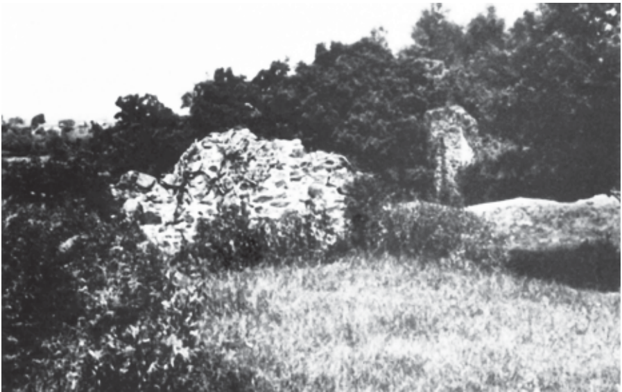
Plate VIII. Wheal Adams. Remains of the buildings around New Engine shaft. The wall in the centre seems to have been an office or a blacksmith's shop. The taller wall, among the trees in the background was probably a whim engine house hoisting from the Engine Shaft situated just out of sight to the right and now hardly visible.
