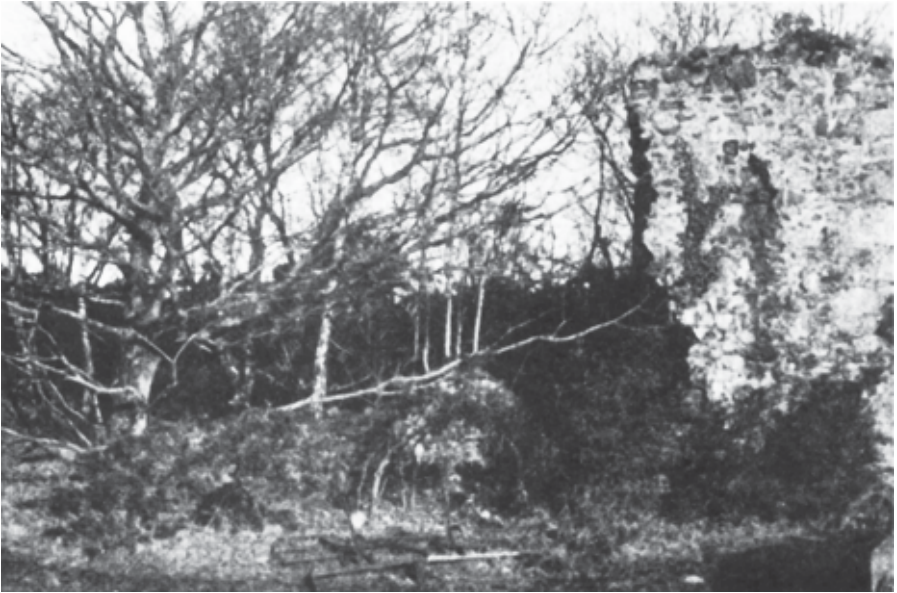
Plate IX. Wheal Adams. A closer view of the remains of the whim engine house. A section of hoisting chain was found by the author (February 1971) half buried in the grass adjacent to this building.
