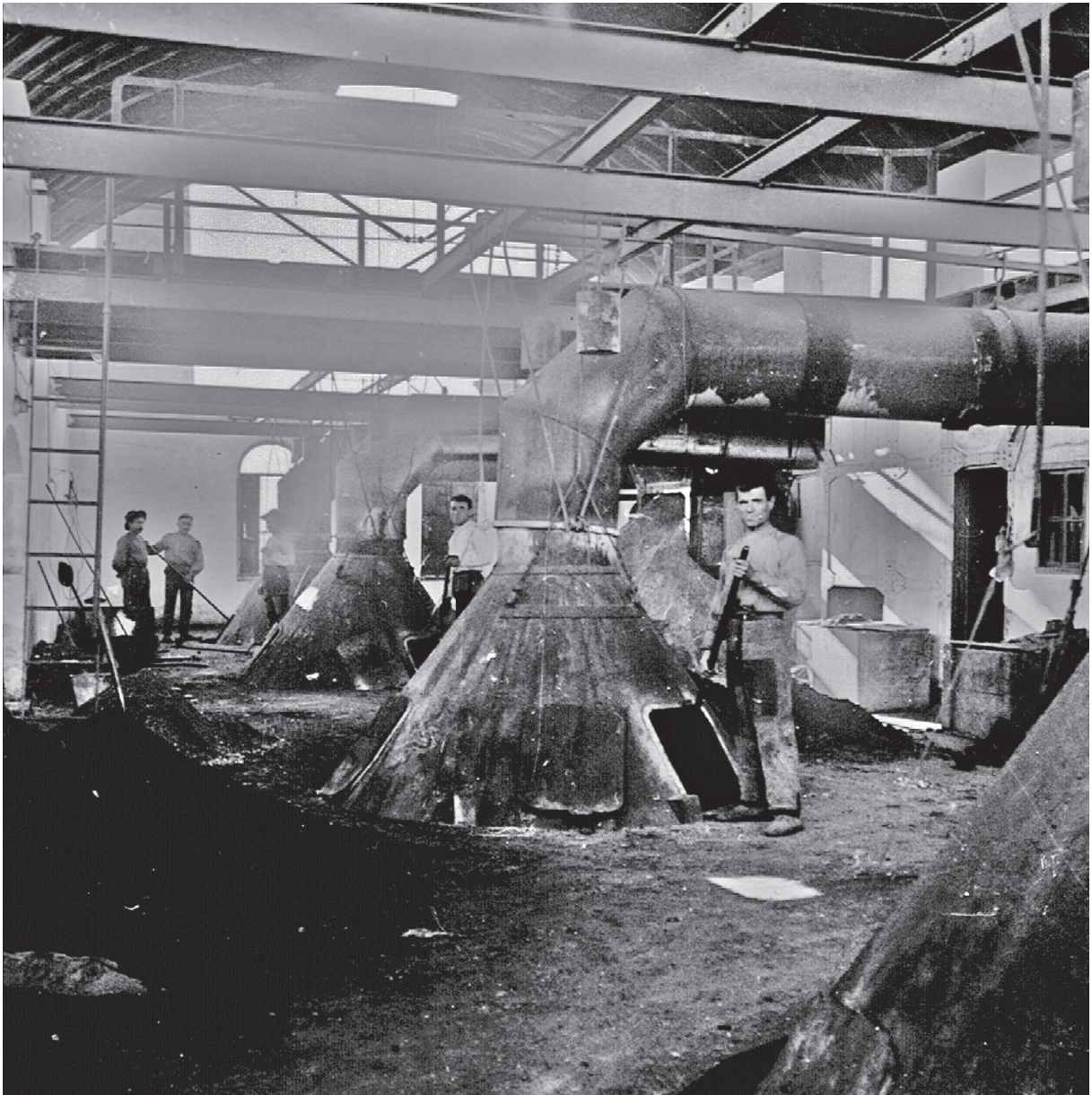
Figure 40. The upper deck of the roasting pots, possibly at La Tortilla, showing the offtake hoods with their charging and working ports. The ducts lead in to vertical rectangular chimneys which can be seen in the background [Colectivo proyecto arrayanes, Linares].
