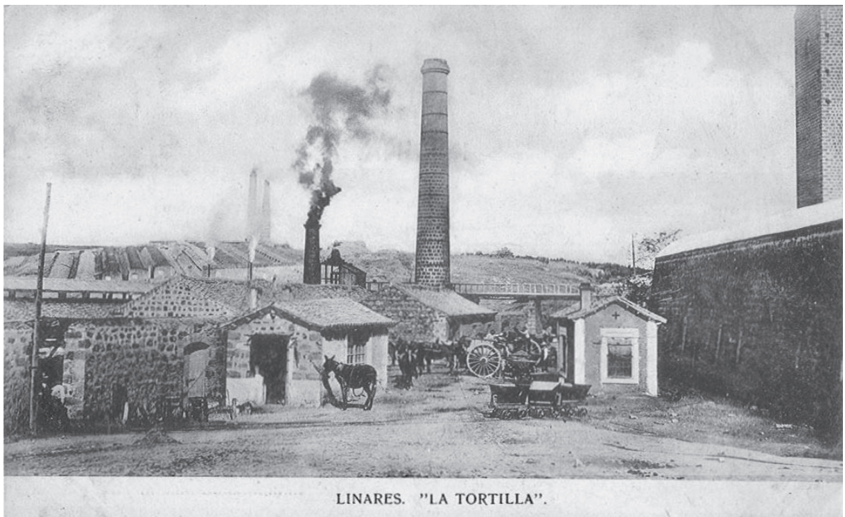
Figure 23. La Tortilla: a view of the lead-works yard. A tramway connected the mine to the works, but donkey carts would have been used for transporting ore from outlying mines. [Author's collection].
