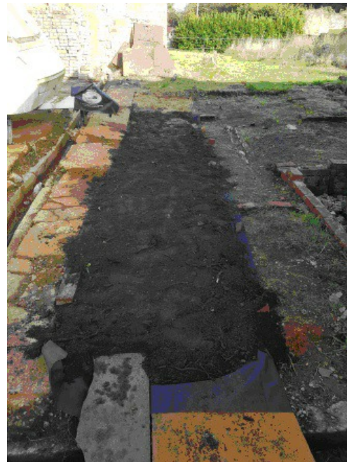
Earth laid on the membrane ready for the contractors
