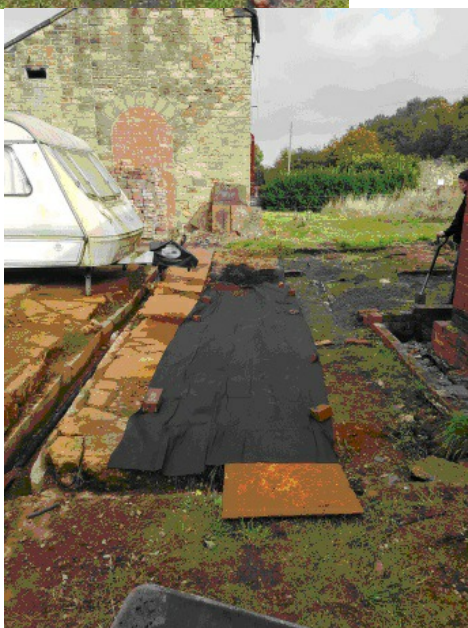
Laying the membrane
