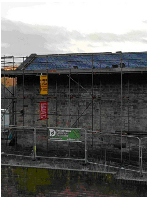
Detail of the restored roof line of the winding engine-house, showing neatly re-laid Welsh slate roof on new battens (photo credit: Glen Sheppard)
