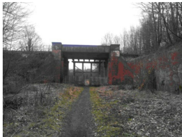
March 2013 – Stead Lane underline bridge
