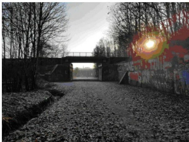
Stead Lane new underline railway bridge, December 2016
