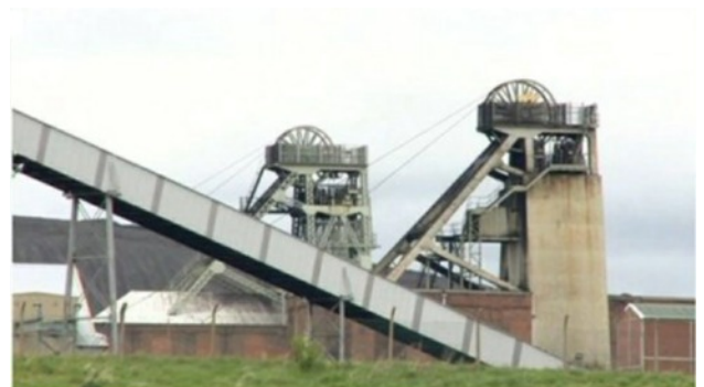
Photo:- A frame structure of Thoresby Colliery
