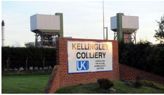
Photo:- Skip winding headgear towers
