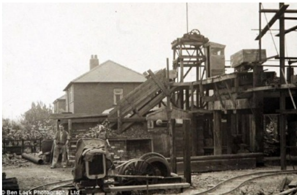
Photo:- A locally made wooden structure (Peggy's mine Wakefield 1940s)
