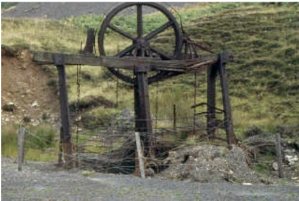
Photo:- Very early wooden structure. (South Wales)
