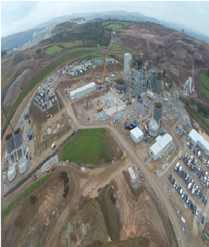
Aerial view of Drakelands Mine.
