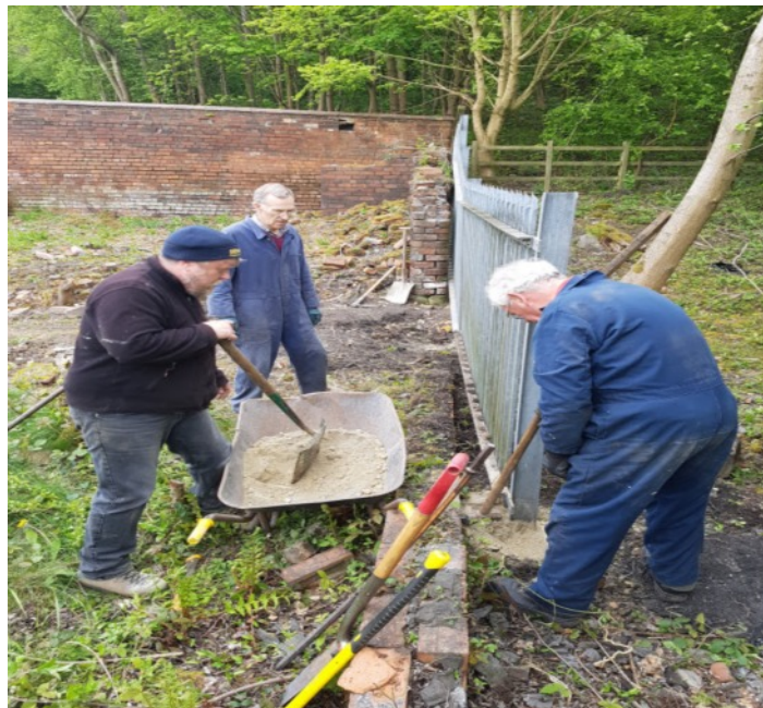
Shovel mix and concreting the fence panels
