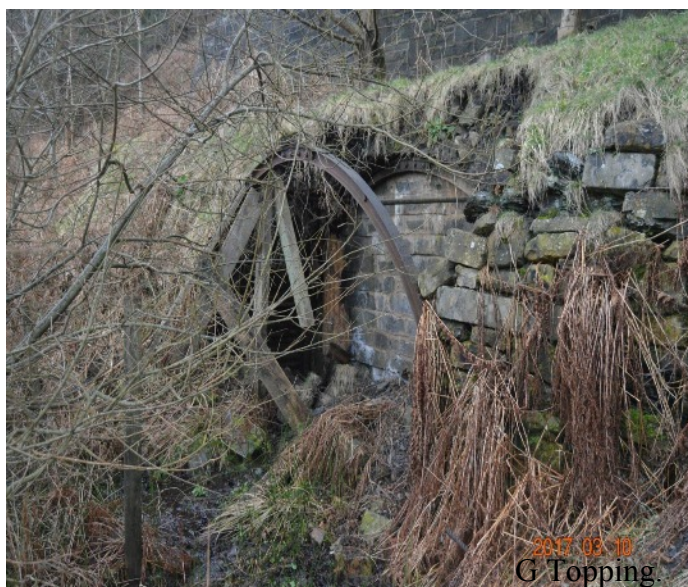
Teak Flow new drift entrance. Upper Mountain Mine.
