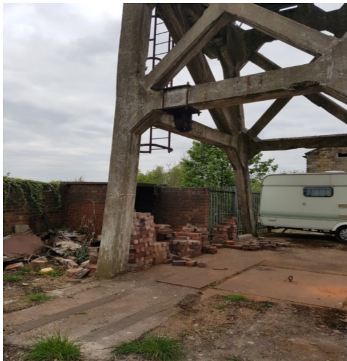
Inspecting the head gear.
