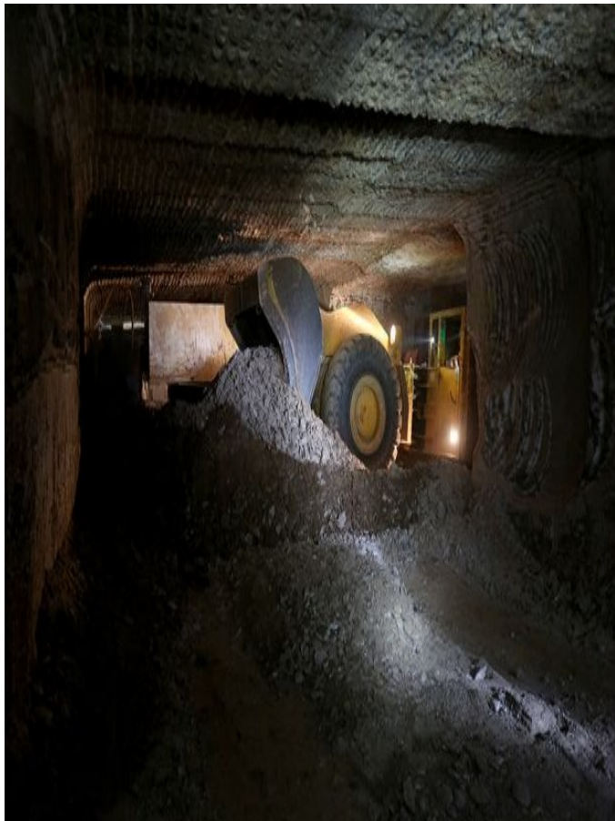
Loading Gypsum underground
