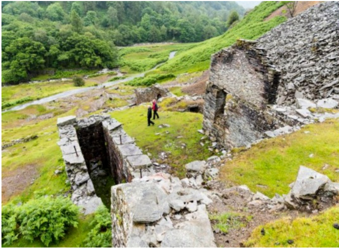
Part of the wheel and wheel well and mill buildings at Penny Rigg.
