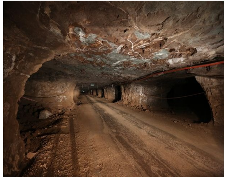
Supporting pillars left in old workings.
