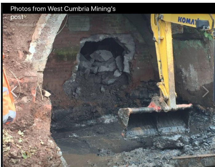
Digger opening up the drift entrance.
