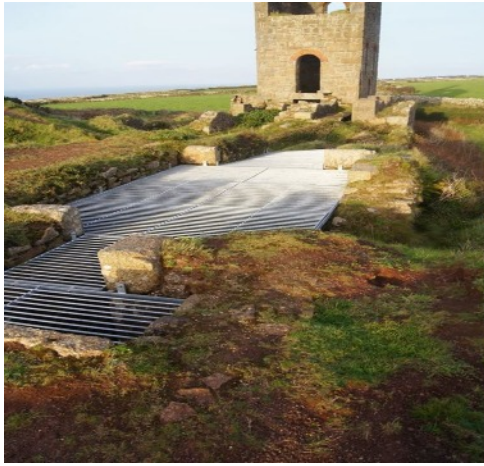
Safety grills fitted at Higher Bal
