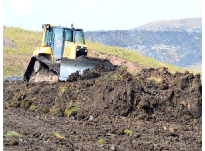
Bulldozer carrying out restoration work at a surface mine in Scotland.
