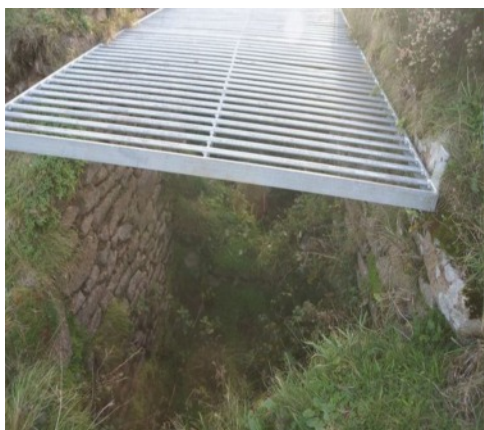
Safety grills fitted at Levant Mine.
