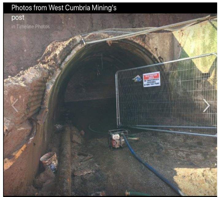
Pumping out residual water in front of the sealing wall.
