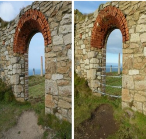
Before and after work carried out at Levant mine.
