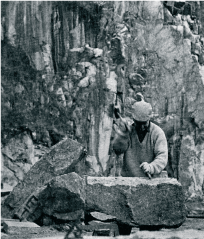
Splitting stone by hand at l'Etacq.
