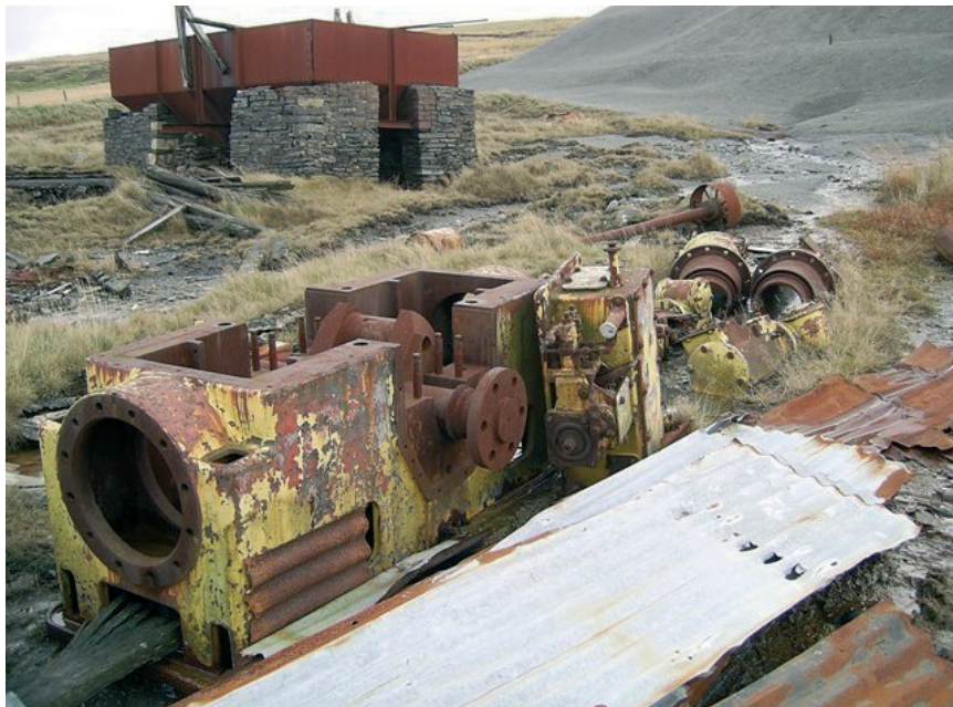
Brush Co. Electrical generating plant and water tank. {2013}
