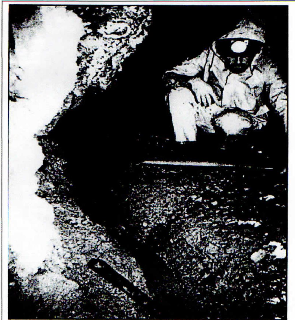
Phil enlarging the drainage channel, Davey's footway shaft end South Drive.
