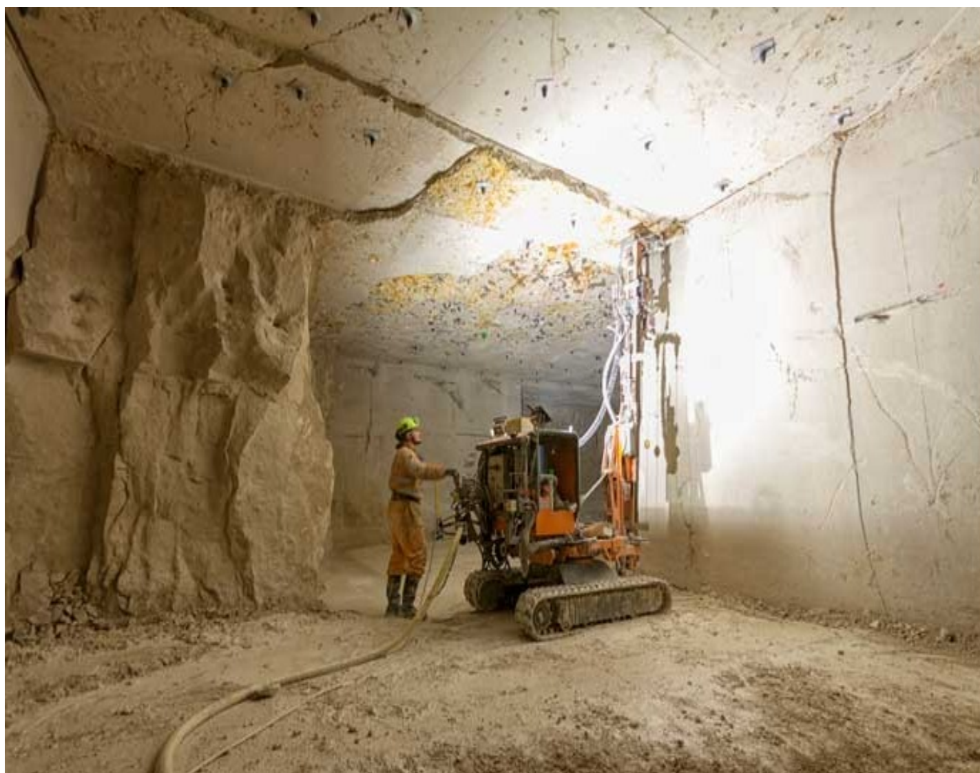
Roof bolting At the Albion Stone Mine.
