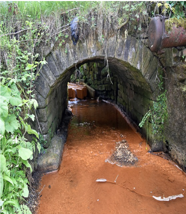
Trawden colliery upper adit. water and capped pipe.
