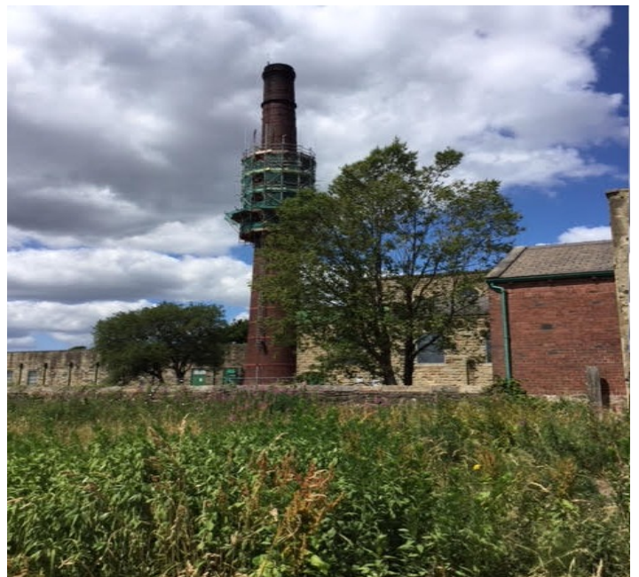
This photo shows the view of the chimney when I went to visit.
