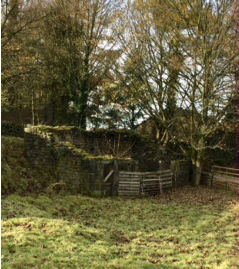
Present day remains of Blacksmiths workshop.
