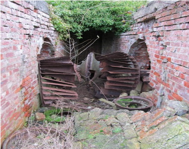
Grinkle Mine Sirocco Fan.
