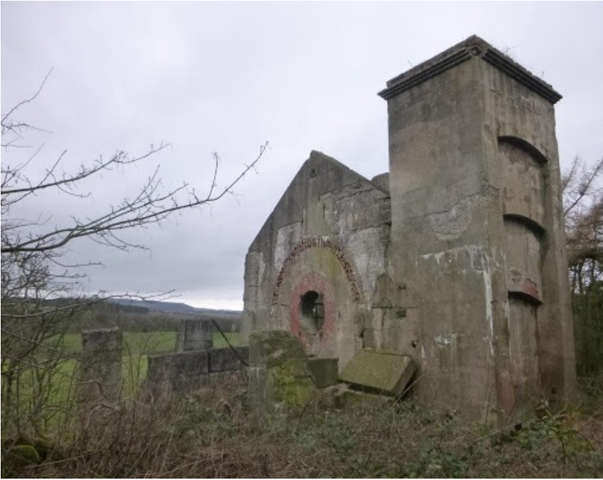
Skelton Shaft Mine, Guibal fan house.
