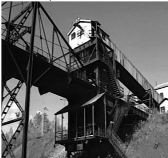
Soudan mine loading gantry.
