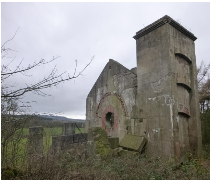
Skelton Shaft Mine fan house.
