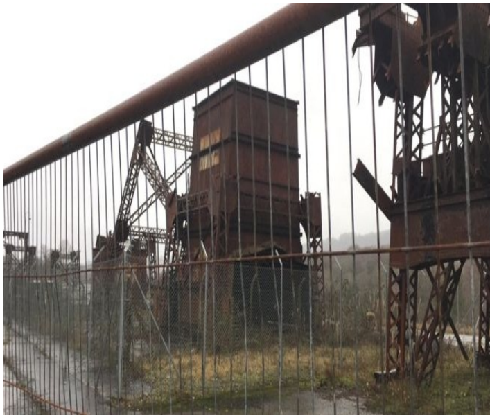
Dismantled winding gear.
