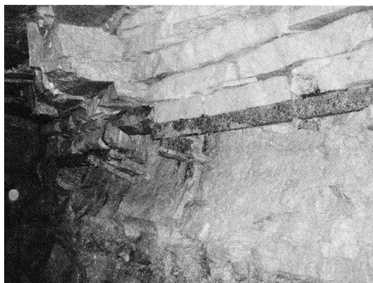
Plate 3. Iron pegs holding up rail.
