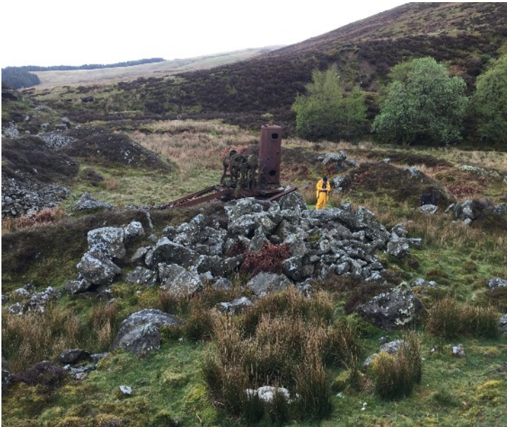
Site layout. About 1 acre in area. Inc. large piles of selected stones
