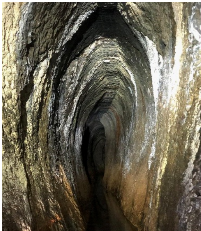
An excellent example of Elizabethan coffin level – part of the Goldscope complex. (MH)
