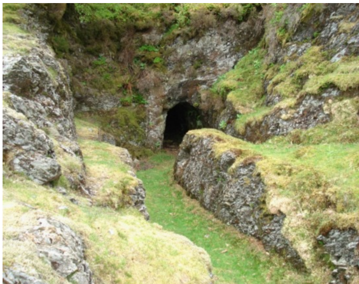
Wheelpit and pump rod adit. GU
