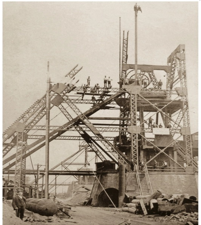
Construction of the head gear 1910.
