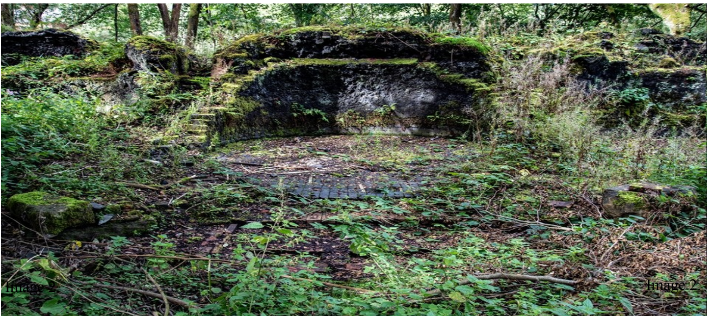
One of the beehive coke ovens {damaged}. Showing the brickwork in the dome, the oven floor and in the fore front the hearth area.
