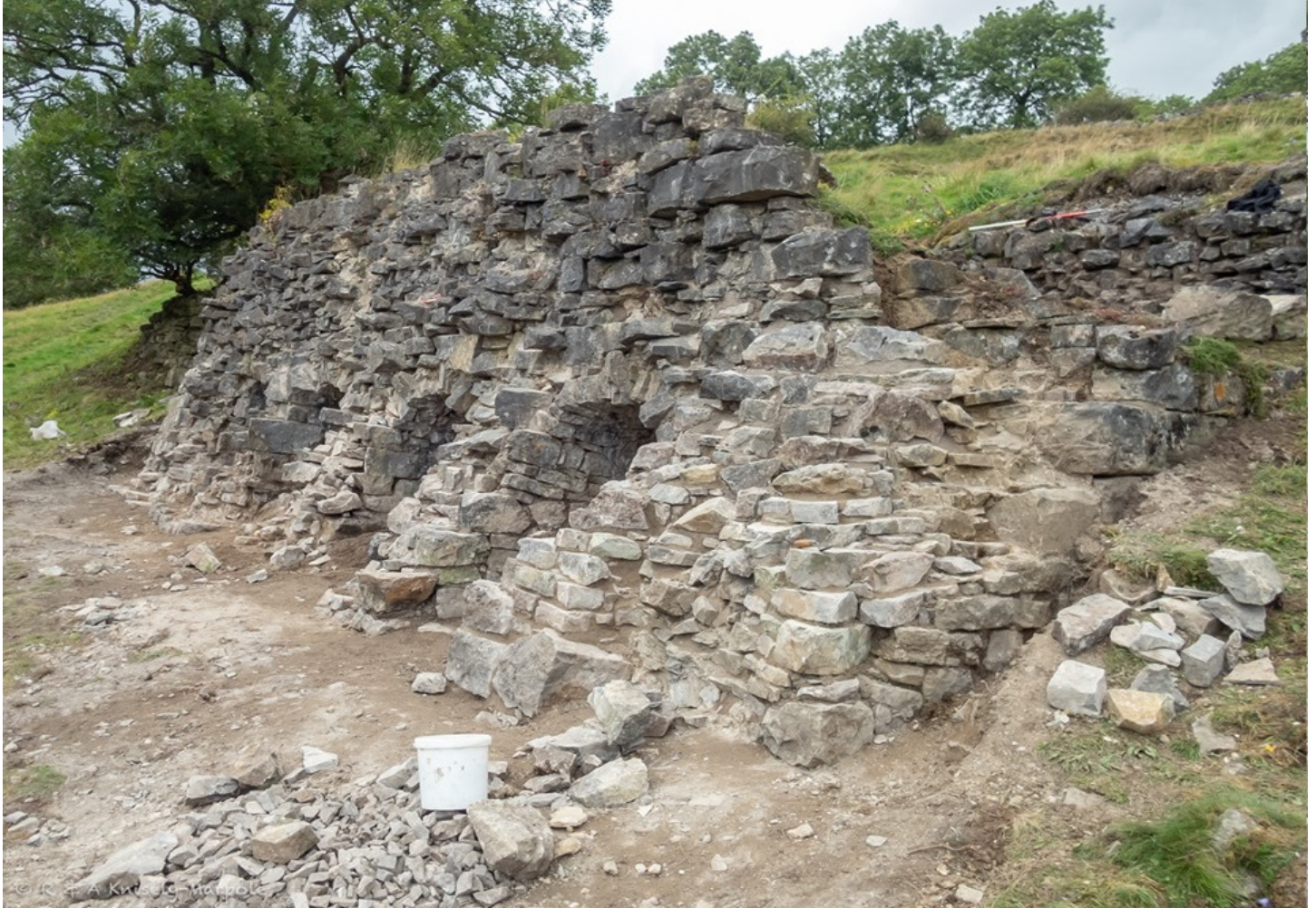
Conservation work taking place at the site.
