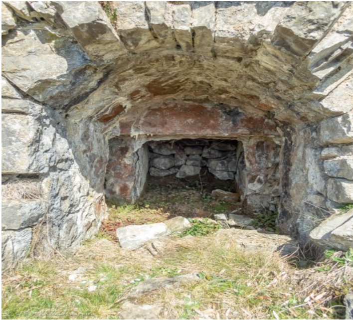
One of the arched tunnels leading out from a chamber of the "ore bin".
