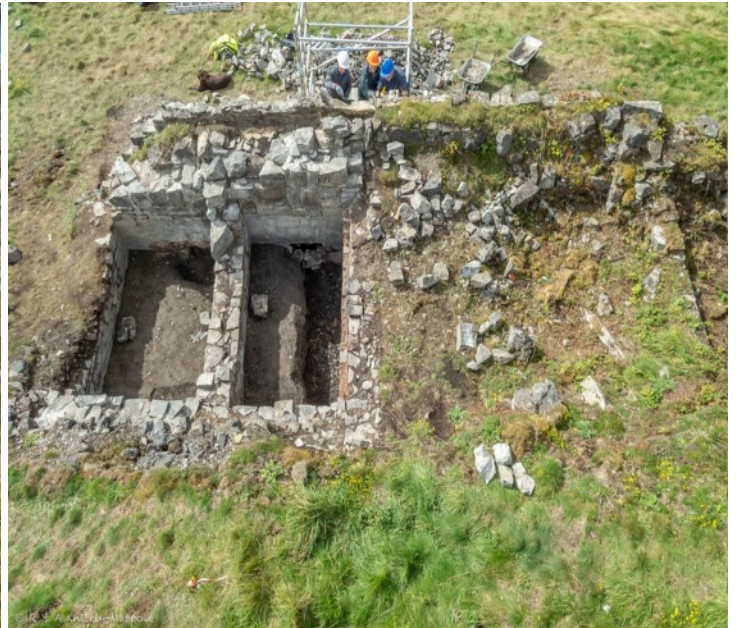
Gradually working our way down to floor level in the bins. Only bins one and two were emptied, as there was insufficient time to do the others {six in all}.
