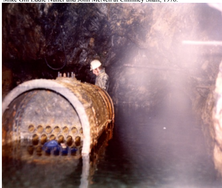
Mike Gill behind one of the multi-tube boilers at Chimney Shaft, 1976.
