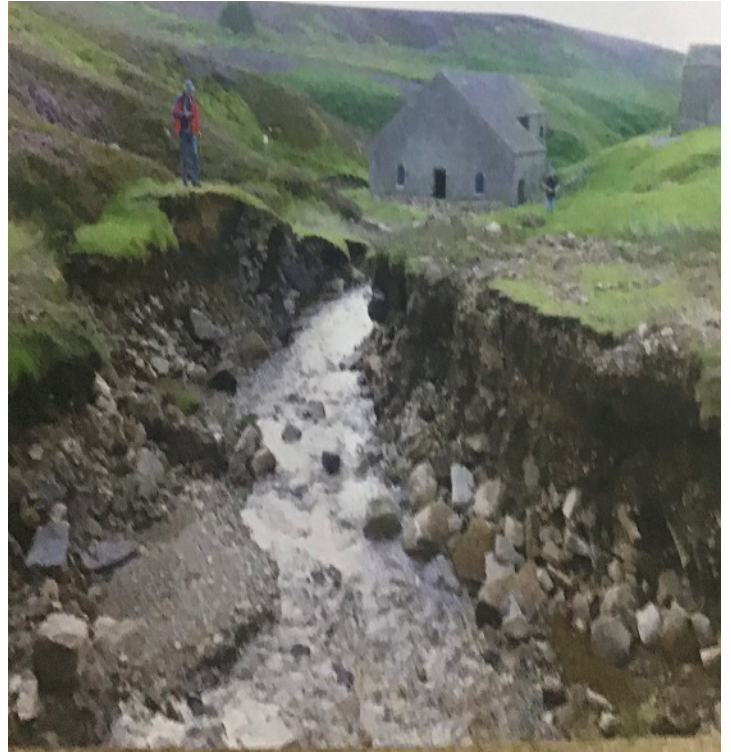
The mill from up the Gill showing flood damage.
