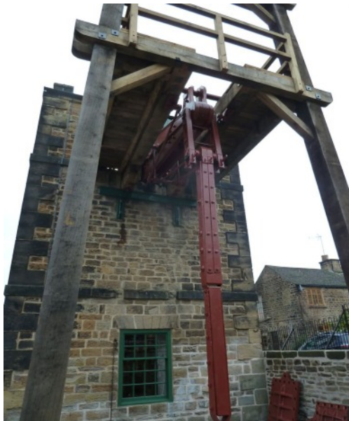
Looking up at the beam and pumping rod.
