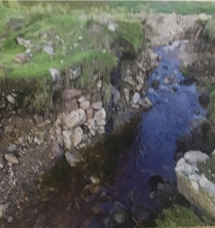
The profile of the lower dam exposed by the floods.
