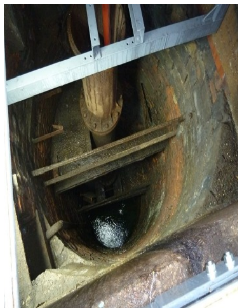
The view down the 100 ft plus pumping shaft.
