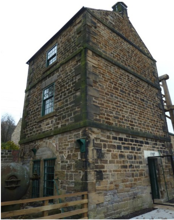
The Elsecar engine house built 1795.
