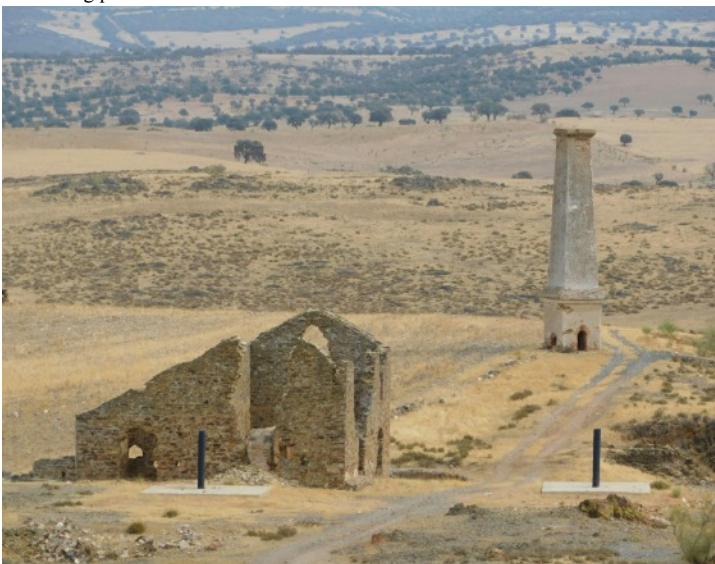
The remains of the Hathorn Davey engine house at La Solana Mine.
