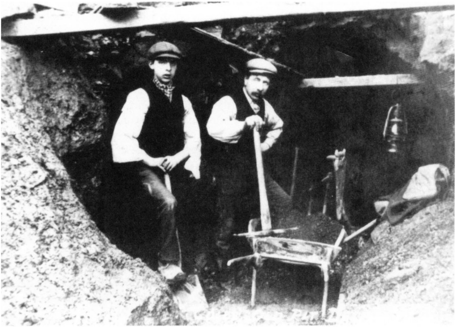
Plate 5. Coll's Old pit, Delph, 1910. An example of a drift mine or 'breast heigh'. (Oldham Local Studies Library)
