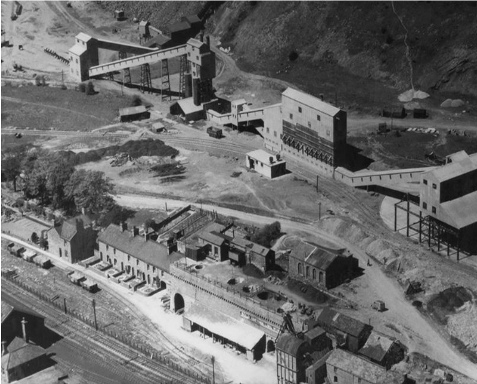
The photo shows the old draw kilns, bottom centre, and the new Horrocksford Lime Co. kilns, top centre.
