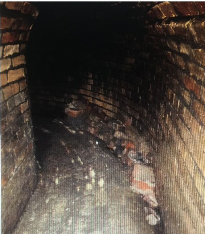
Boiler flue connection to Chimney
