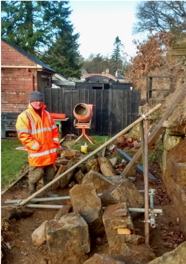
North York Moors Railway collapsed wall repair.
