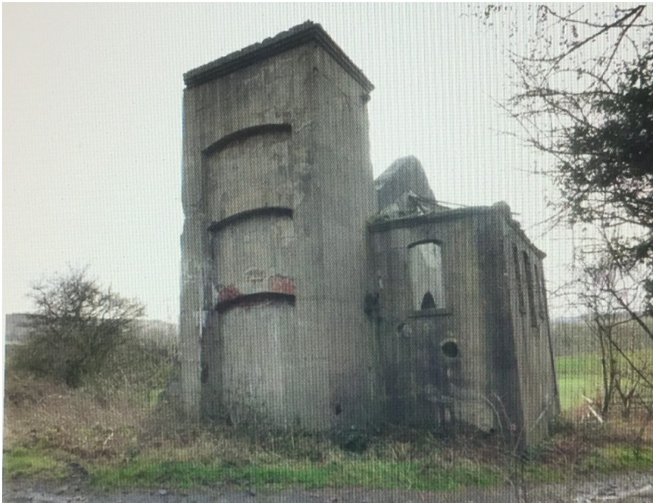
Skelton shaft mine Guibal fan house.
