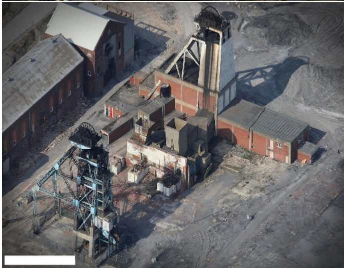
3 Drone photographs of Hatfield pit top area
