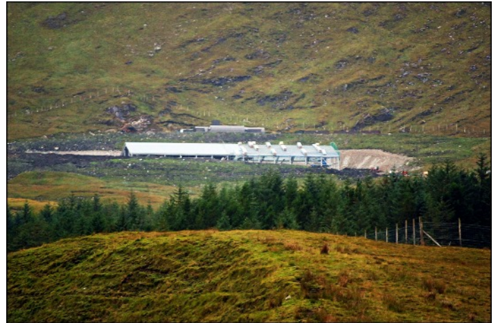
Cononish mine in a view from the West Highland Way In a view that locates the process plant.
