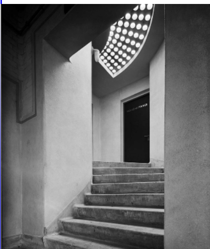
Modernists design clearly visible at Betteshanger Colliery Pithead baths entrance Kent. {1930s}
