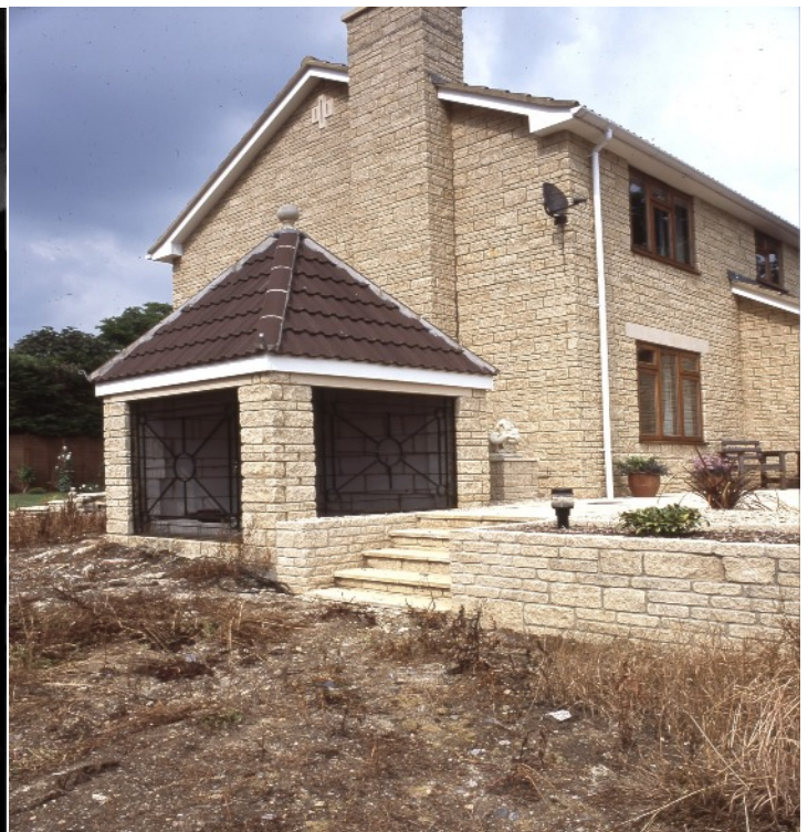
When the surface was re developed, the developers discovered that the ventilation shaft still in use. So they incorporated it in to a gazebo type structure attached to one of the property's.
