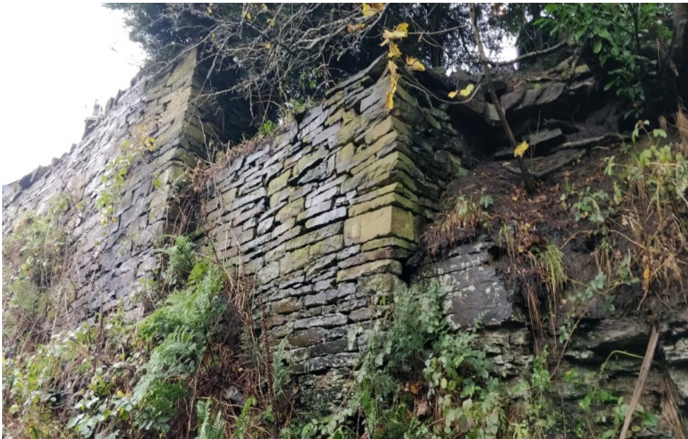
Bridge abutments for tramway over the road at Hall Fold.
