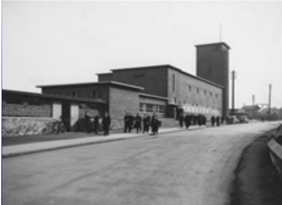
Miners' welfare and pithead baths buildings at Manvers Main Colliery, South Yorkshire. {1940s}
