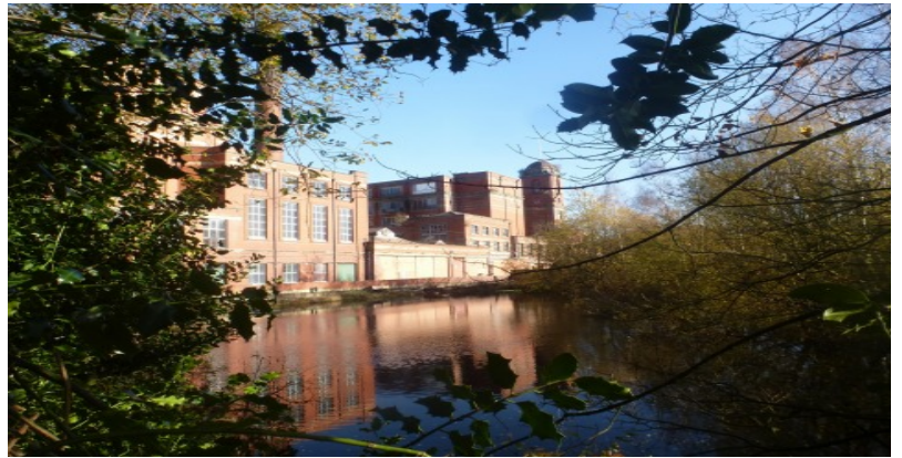
No.1 engine house and mill in the back ground. The central boiler house that contained 7 Lancashire boilers and chimney. No.2 engine house and mill on the left with the lodge in the foreground.
